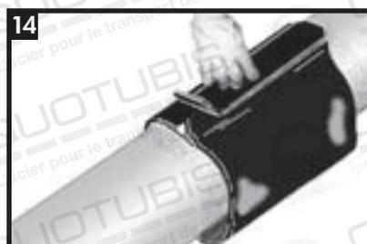
Remove any release liners from the closure. Centre the closure on the overlapping sleeve. Press down firmly.
